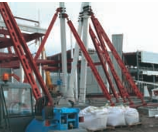
Raking Megashors propping steel columns
