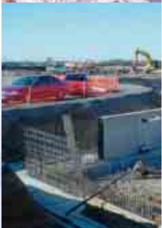
Client: Paveways Project: Bell Vista Residential Canal, Caloundra, QLD
