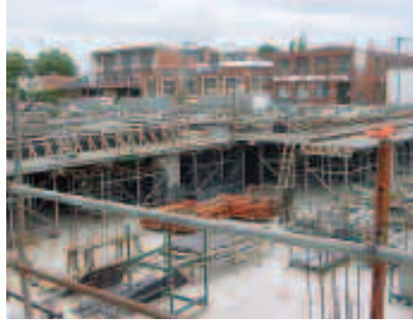
Airodek panels on Rapidshor support.
