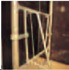
Assembly gates are used to provide stability and panel spacing
