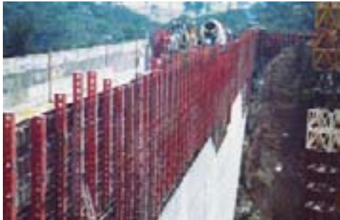
Rapid Ply, Molonglo Dam, Canberra
