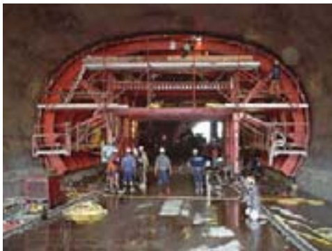
Special Formwork, The Buranda Tunnel, Buranda, QLD
