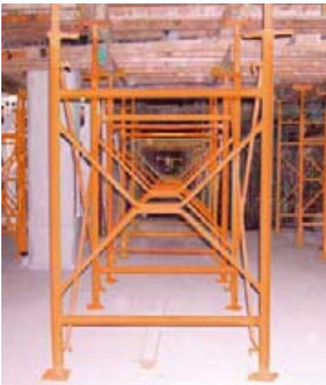
Strongshor, Bent Street Apartments, Adelaide, SA
