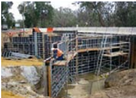
Kilt Brook Bridge, WA
