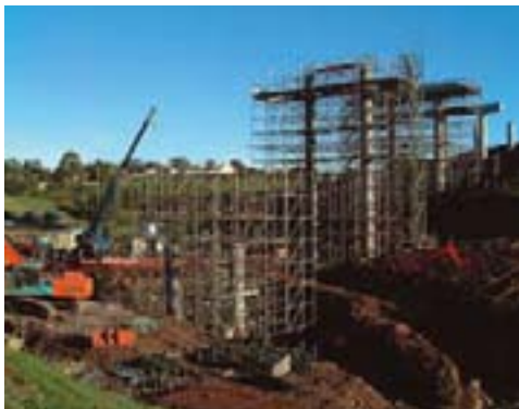
Rapidshor, Grant Creek Bridge, Adelaide, SA
