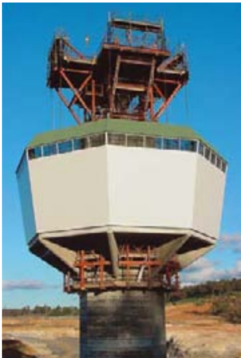
Harvey Dam, Harvey, WA
